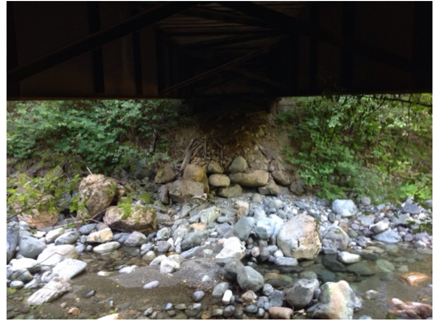
Left Bank Abutment when facing downstream
