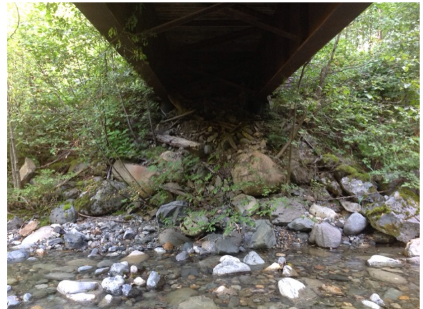
Right Bank Abutment when facing downstream
